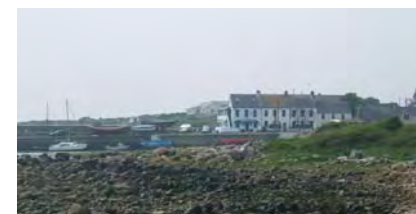
The existing terrace along Pier Road displays an important contextual relationship with the pier and is one of the few remaining parts of the village that has a vernacular streetscape.
