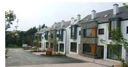
New housing developments tend to reflect an urban character as a result of the building forms, materials and densities applied in new estates.
